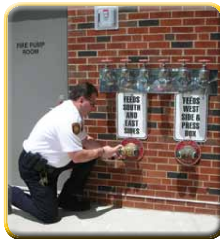
Bruce McAvoy installing Knox® Locking FDC plugs at Kinnick Stadium
